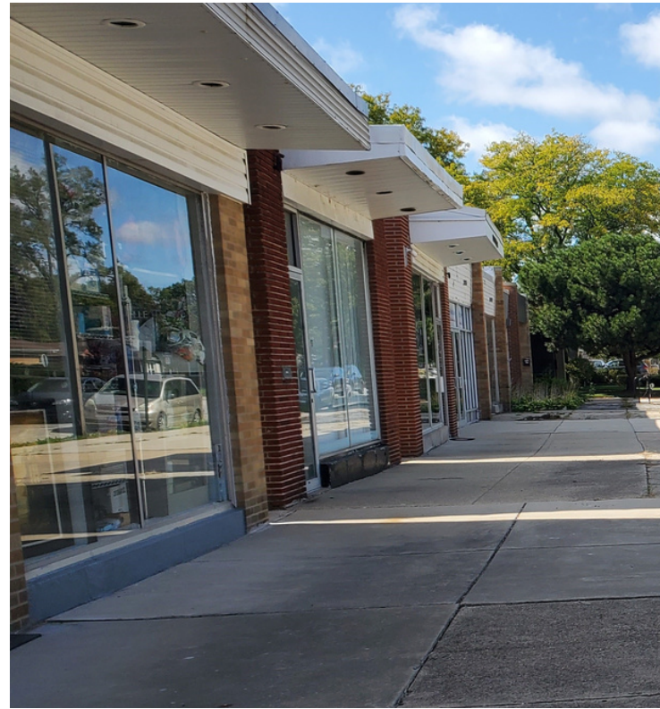
Vacant store fronts with wide, unused, concrete plazas
